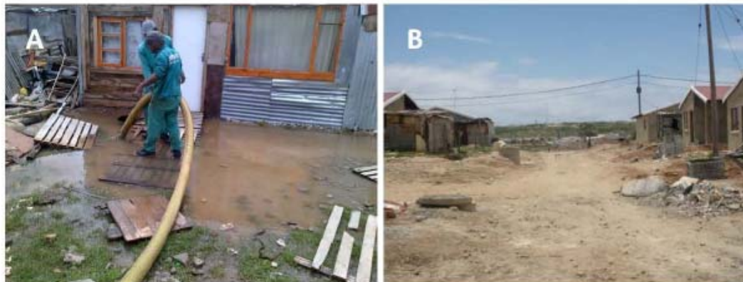
Fig. 3. Municipality pumping off the water in front of the informal settlement house and B) Area with new building, built on flood plain (All photographs were taken during fieldwork observation).
